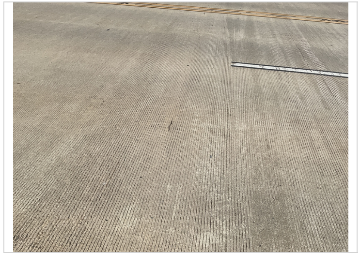
Deck has sealable transverse cracks
