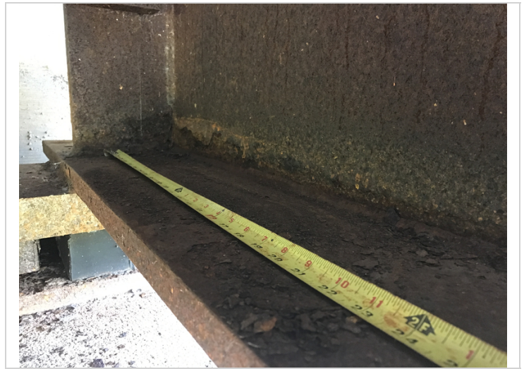
Bent 4 beam 8 laminating rust on inside of beam end
