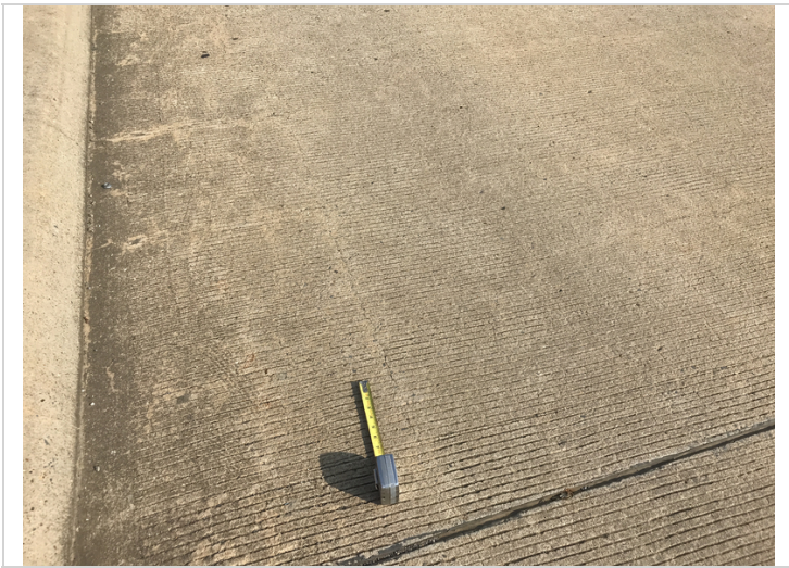
Span 3 longitudinal crack up to 0.015"
